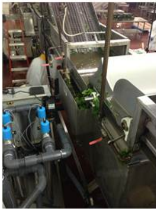
Wash Water Tank
