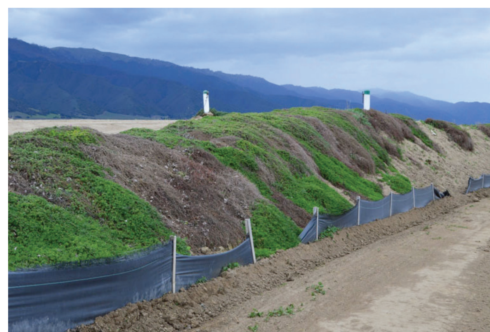
Figure 2. Traditional silt fence exhibiting wind damage, originally installed to exclude frogs and other wildlife from the growing environment.
