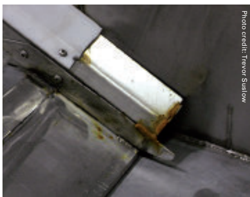
This new line has a clear design flaw, showing junction gaps and trapped crop tissue still present after cleaning. It would be considered a safe harbor site for Listeria.
