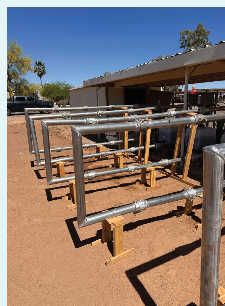
Figure 1: Aluminum Irrigation Pipe Loop
